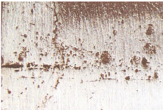
Figure 7. Pitting Corrosion of Stainless Steel Tubing
